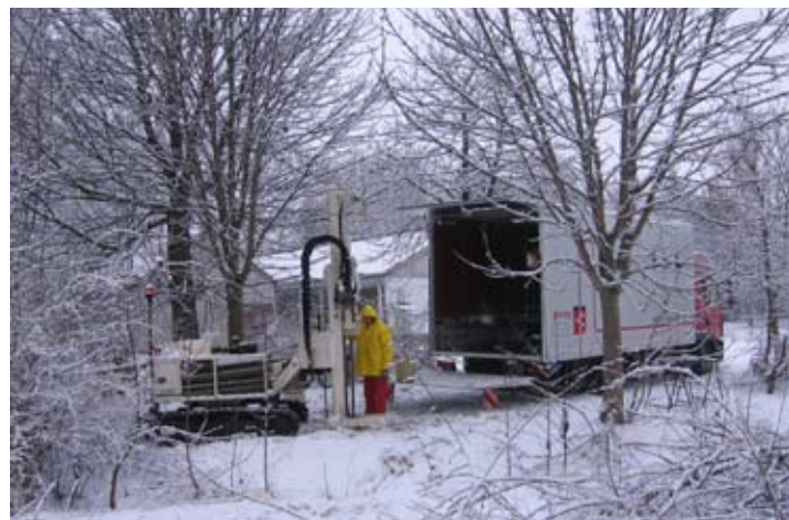
At a site in eastern Hungary, the geo-log team experienced temperatures below -10° C while performing MIP logging, groundwater and soil sampling.
